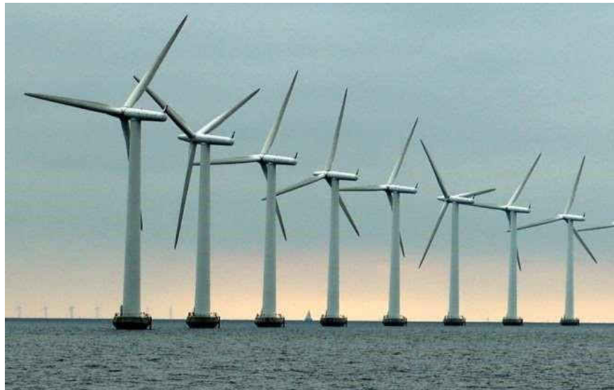
Fig2.2.2 Off-shore wind farm
